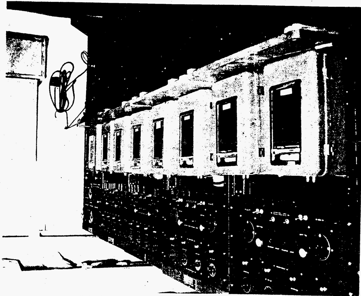
Mark 42 Mod 6 degaussing range control system installed in Surfbird .
